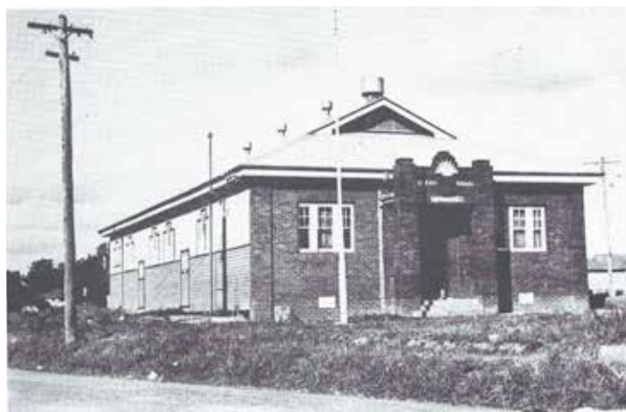
1936 - ANZAC Memorial Hall, built in 1935 Junction of Old Castle Hill and Old Northern Roads
