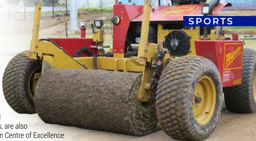
Turf being laid at Kellyville Memorial Park. Picture: Courtesy Western Earthmoving
